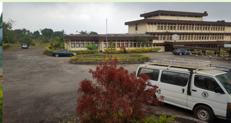
Back view of PAID-WA Buea main campus
