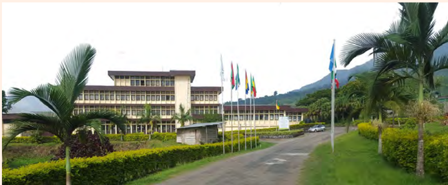
Front view of PAID-WA Buea main campus
