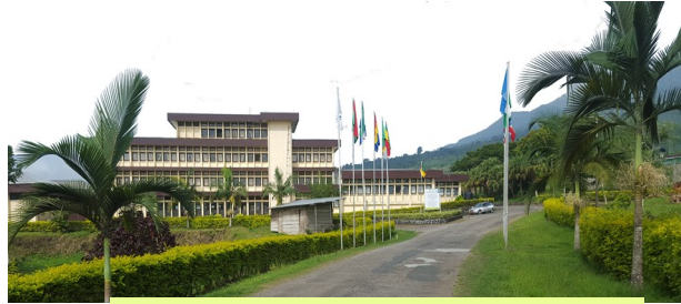
Front view of PAID-WA Buea main campus
