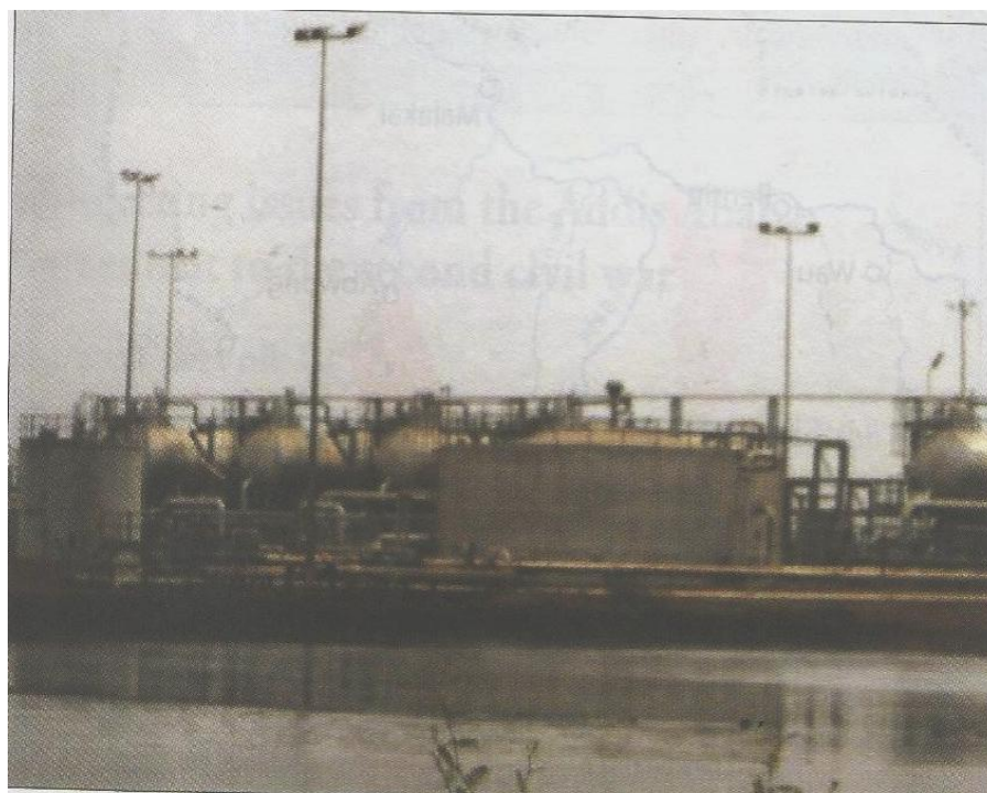
Figure 2.1 Oil Storage Facility in Bentiu, Unity State, Republic of South Sudan (National Ministry of Petroleum & Mining).
