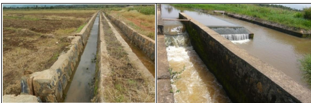
Figure 4. 4: Canals to enhance water distribution in the rice fields
