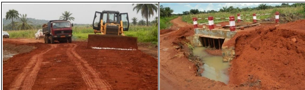
Figure 4. 3: Road Maintenance and Bridge-Bali Road June 2015
