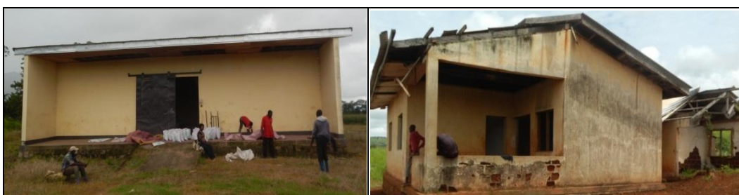
Figure 4. 5: Warehouse and dilapidated sector resident under repairs. July
